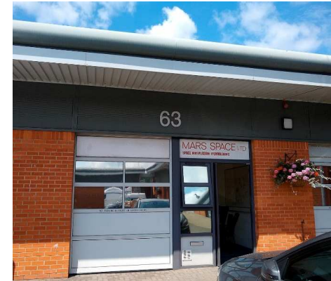
Offices Basepoint, Southampton
