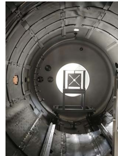
Internal view from end cap
